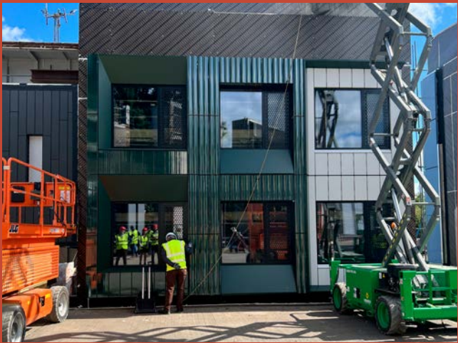
Off site façade mock up to ensure performance requirements were met before sign-off for construction.
