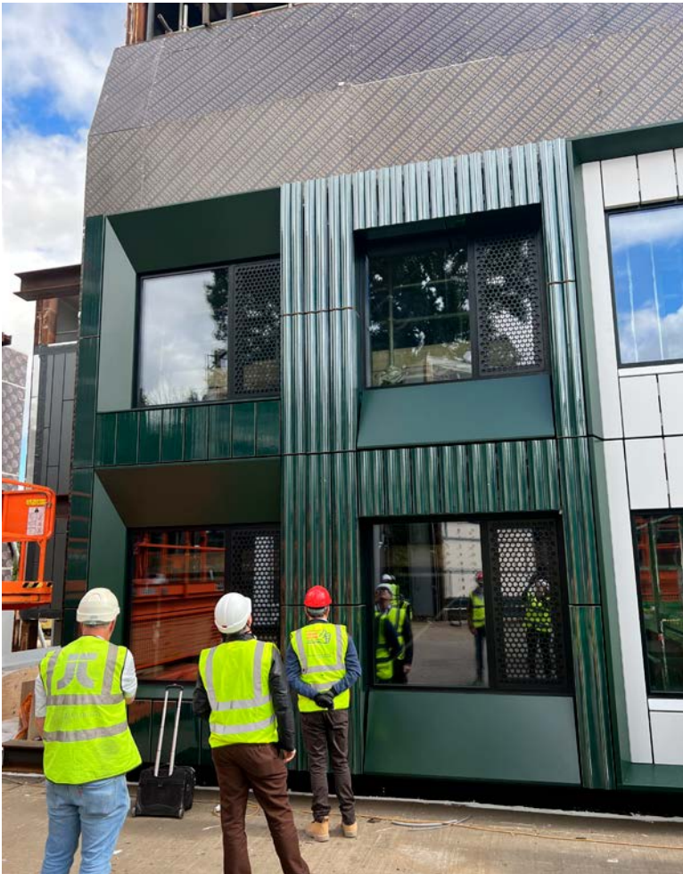
Façade mock-up for a dual review on visual and performance due to tight project programme
