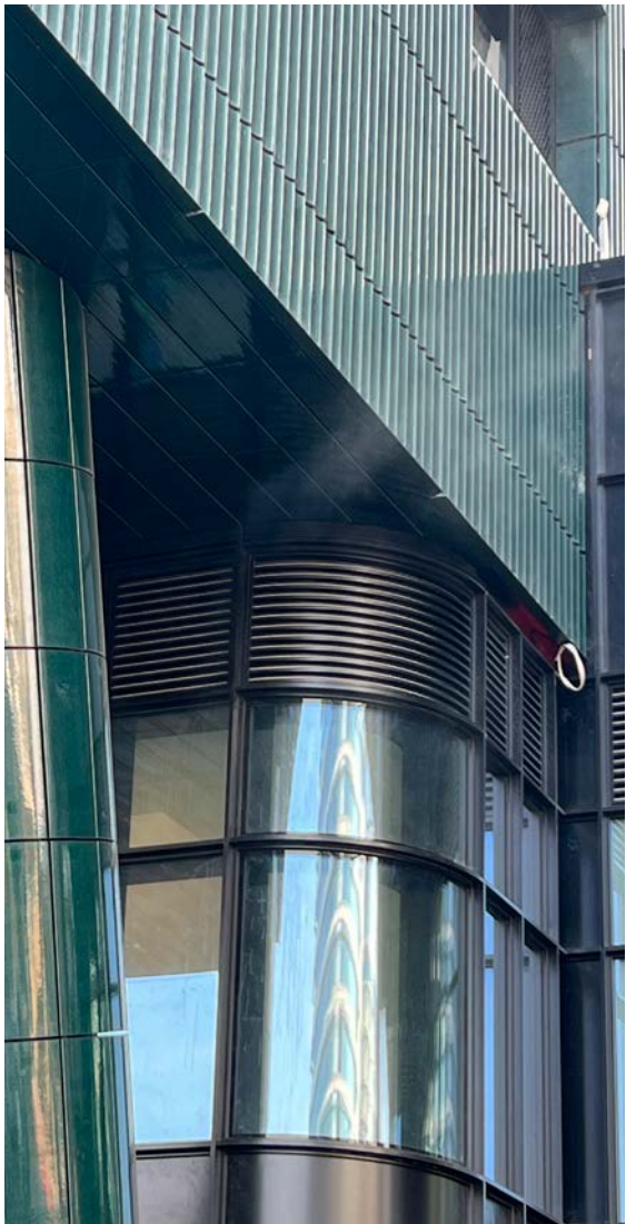
Smoke machines in action Observation of leakage through louvers at podium level
