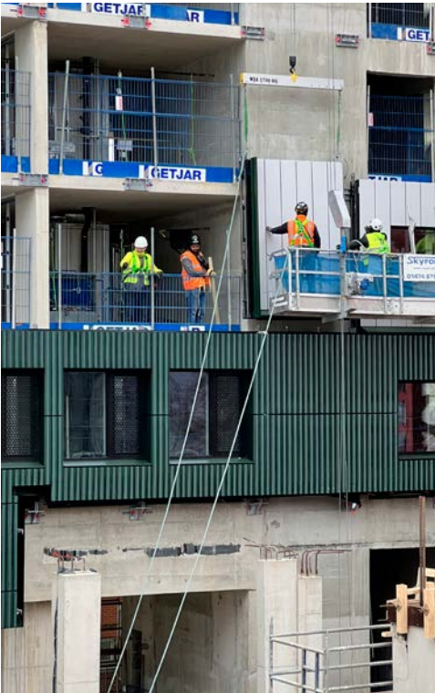
Panel installation requiring 4-5 builders for accurate fitting
