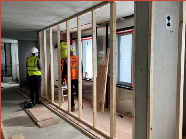
Onsite façade panels testing involved setting up testing rigs around 8 selected areas to measure the as-built leakage, ensuring delivery and installation did not compromise the airtightness performance of the design.
