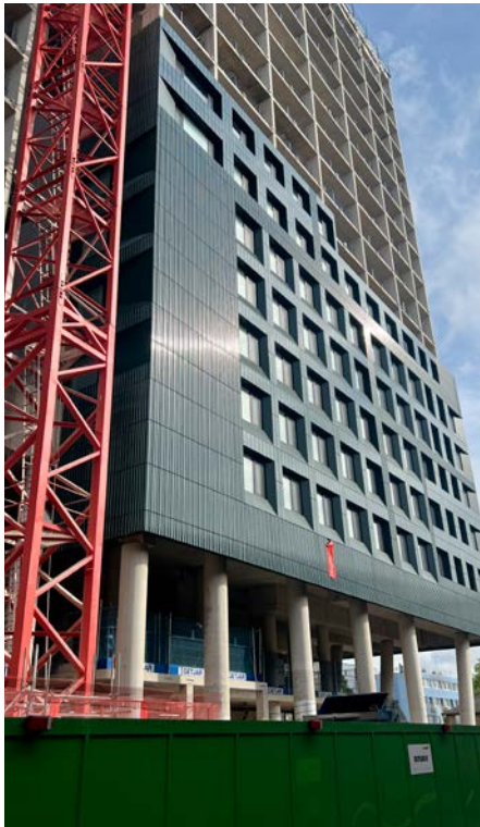
Unitised panel assembly in progress
