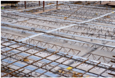
Preparation of reinforcing rods and post tension bars
