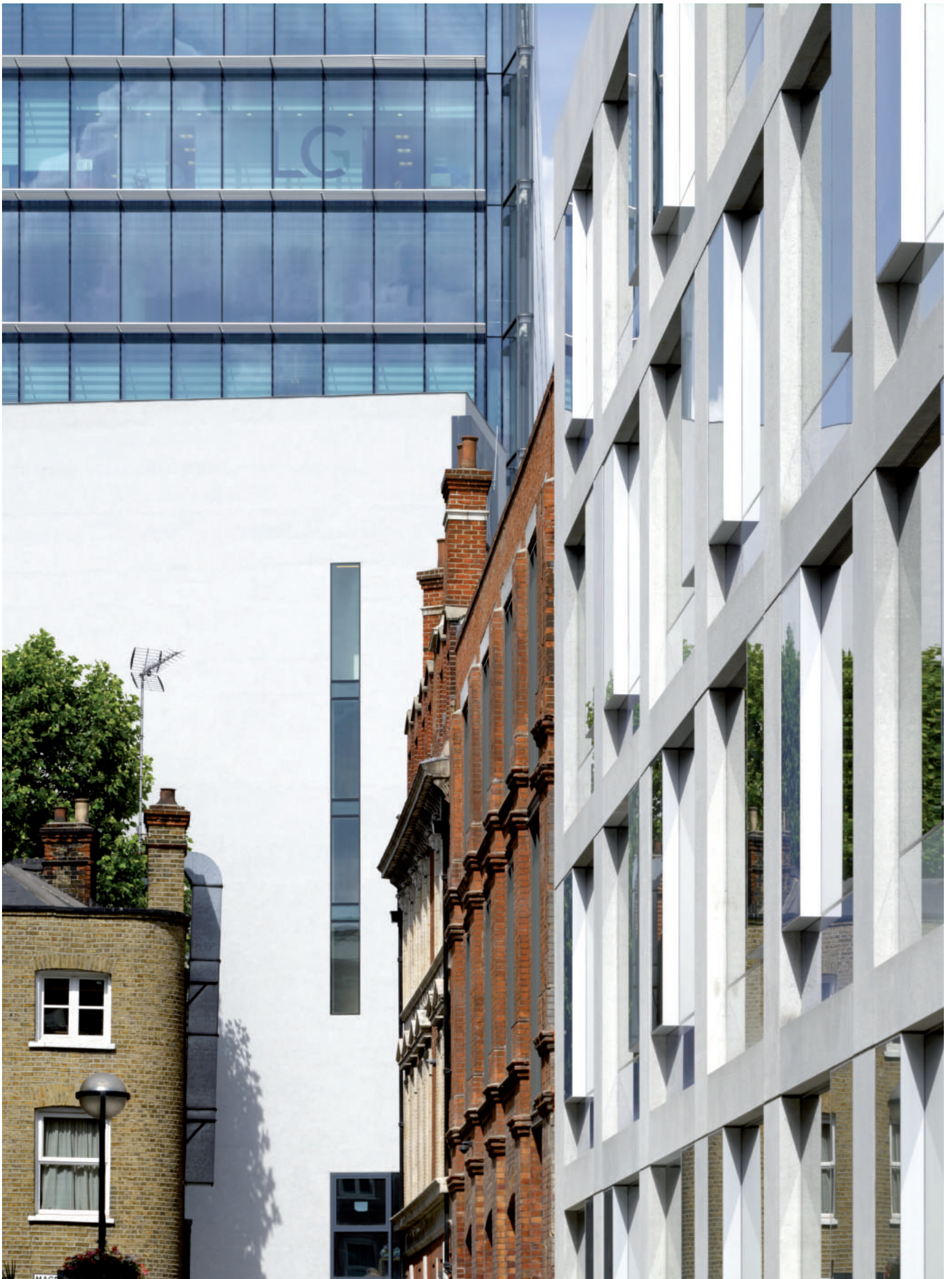
View from Shand Street showing junction of old and new (More London in the background)
