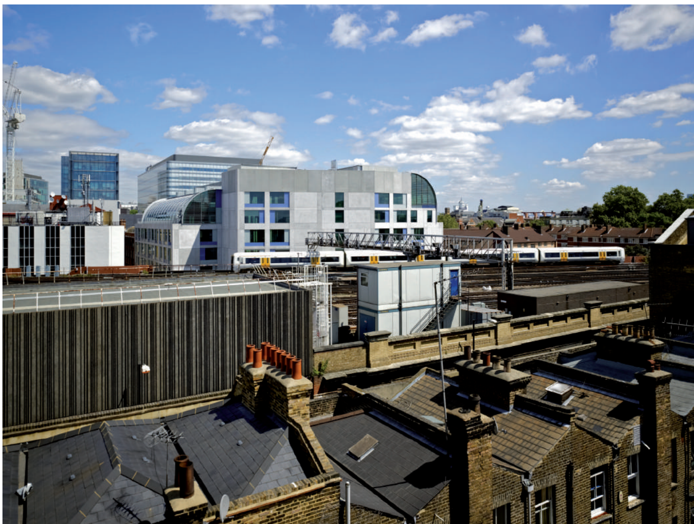
South façade overlooking train viaduct
