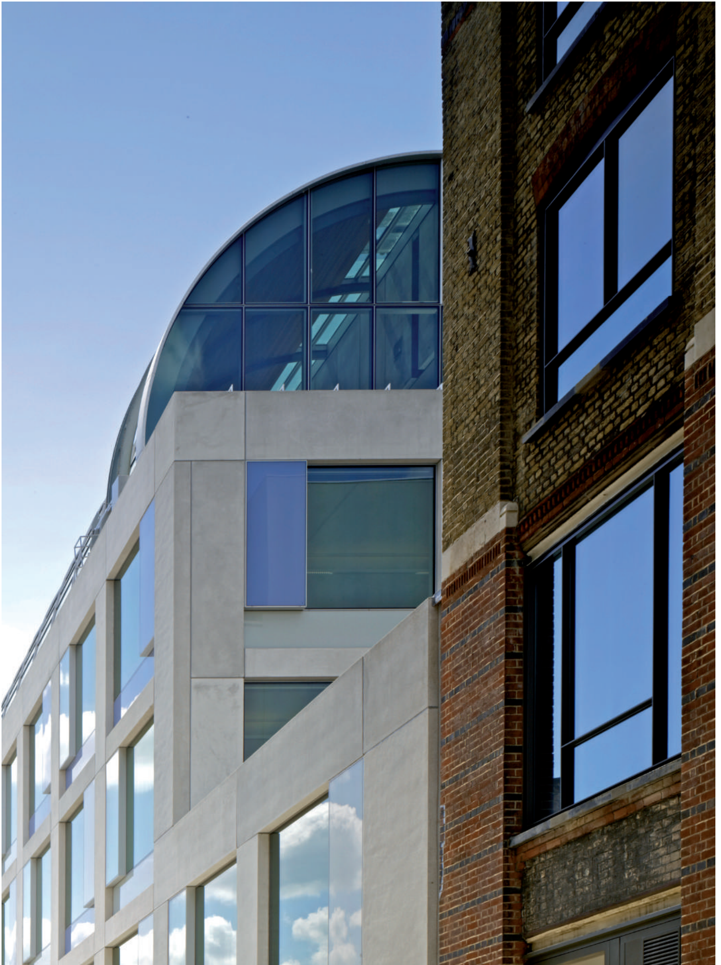
Detail view in Barnham Street - new façades reinterprets existing; barrel vault to top floors
