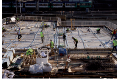
Formwork table to support precast soffit
