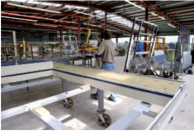
4.05 Unitised cladding in construction
