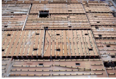
Formwork table to support precast soffit
