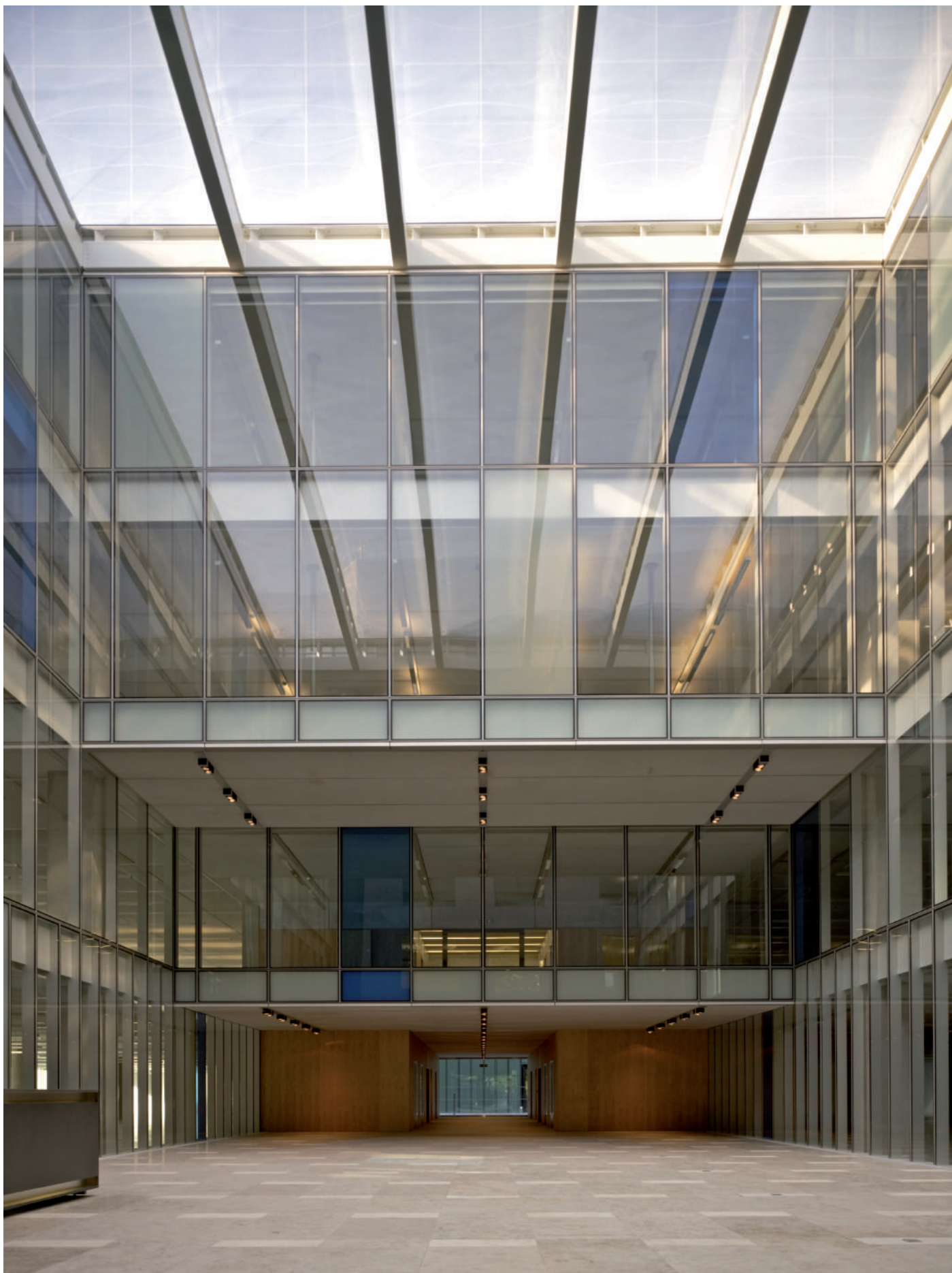
Atrium space with ETFE roof
