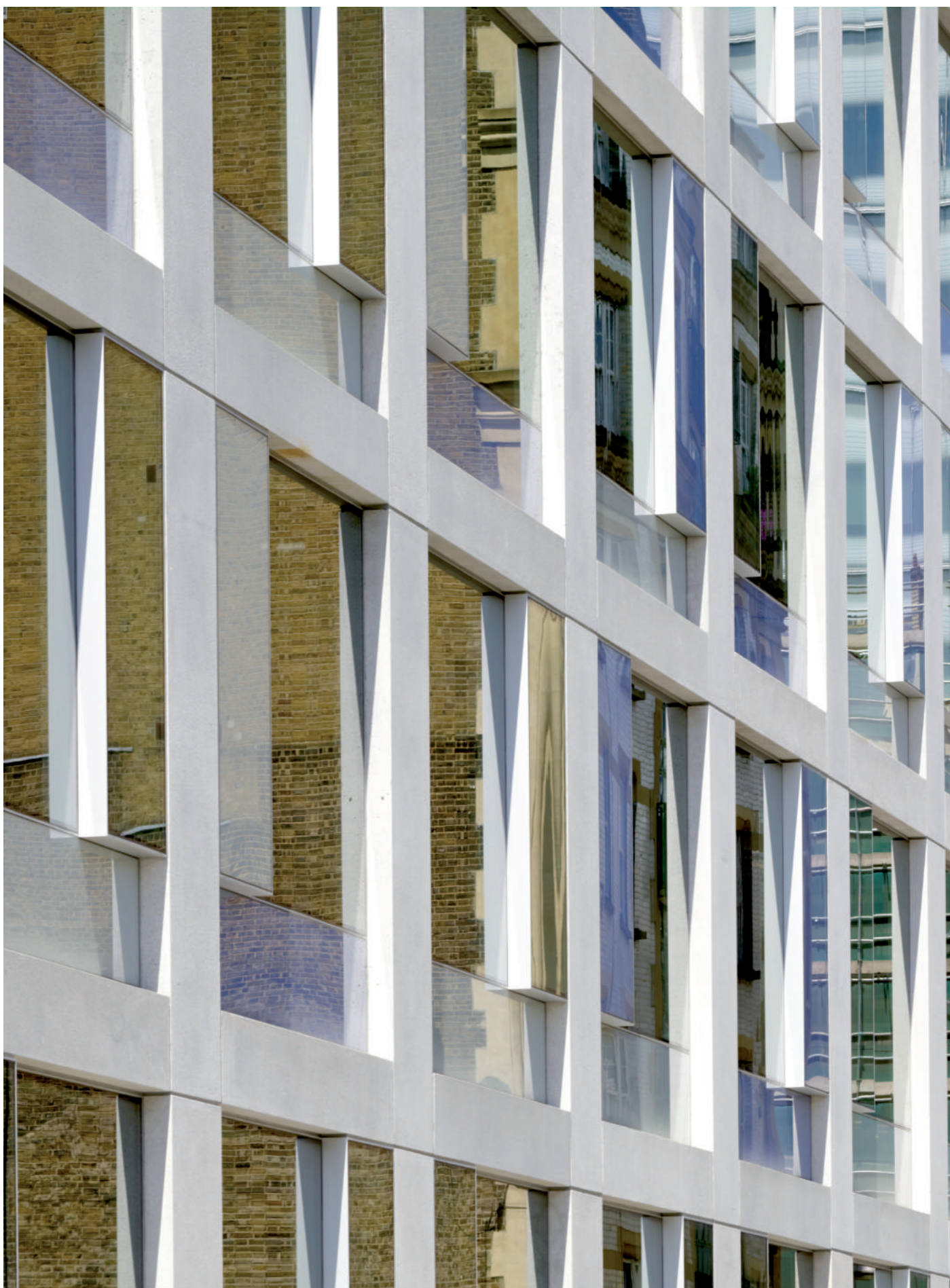
Barnham Street façade - Punched windows with articulated projecting bays, in precast frame
