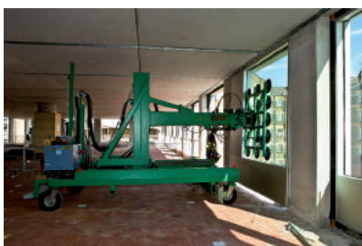
Installation of unitised cladding
