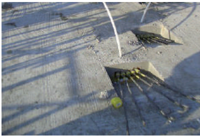
Post tensioning of slab
