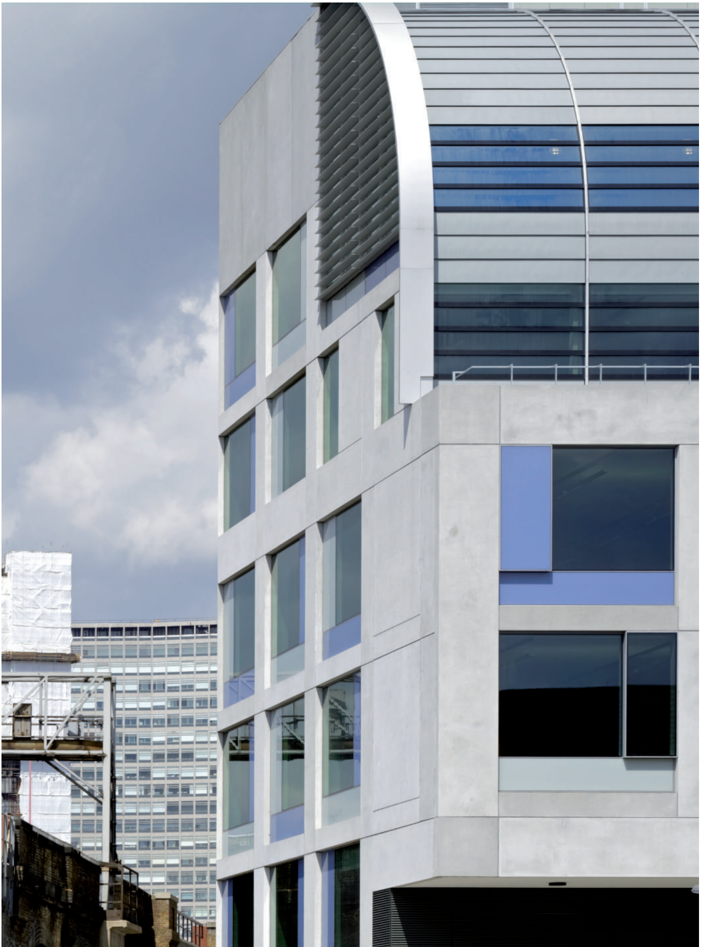
South façade overlooking railway viaduct
