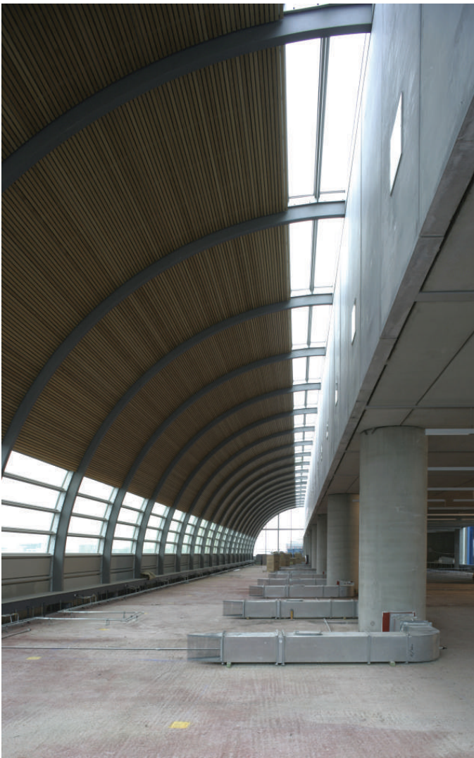
Self finished prefabricated components for repetition, integrated structure and services
