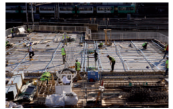
Preparation of reinforcing rods and post tension bars
