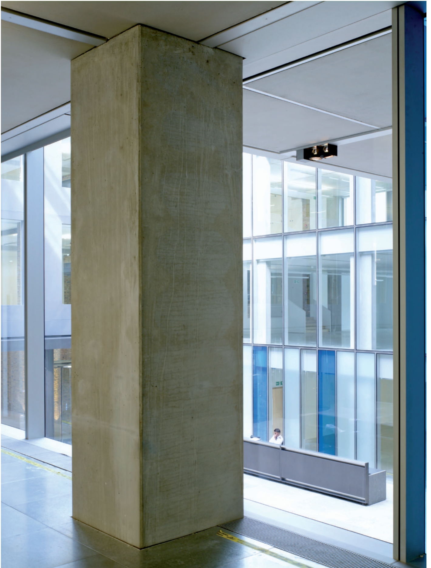
Precast concrete column with atrium behind
