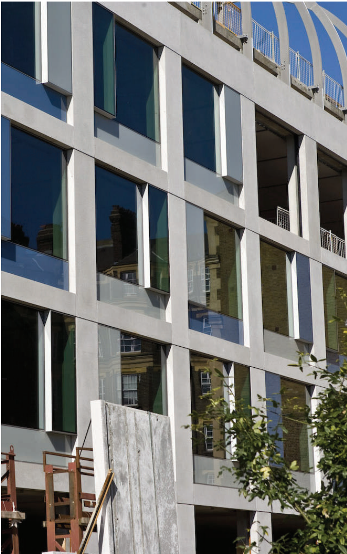
Assembly of pre-fabricated components
