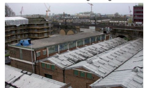
View south over site before demolition
