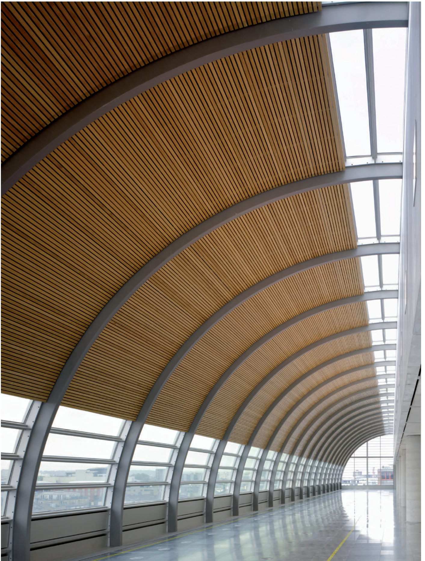
Barnham Street barrel vault
