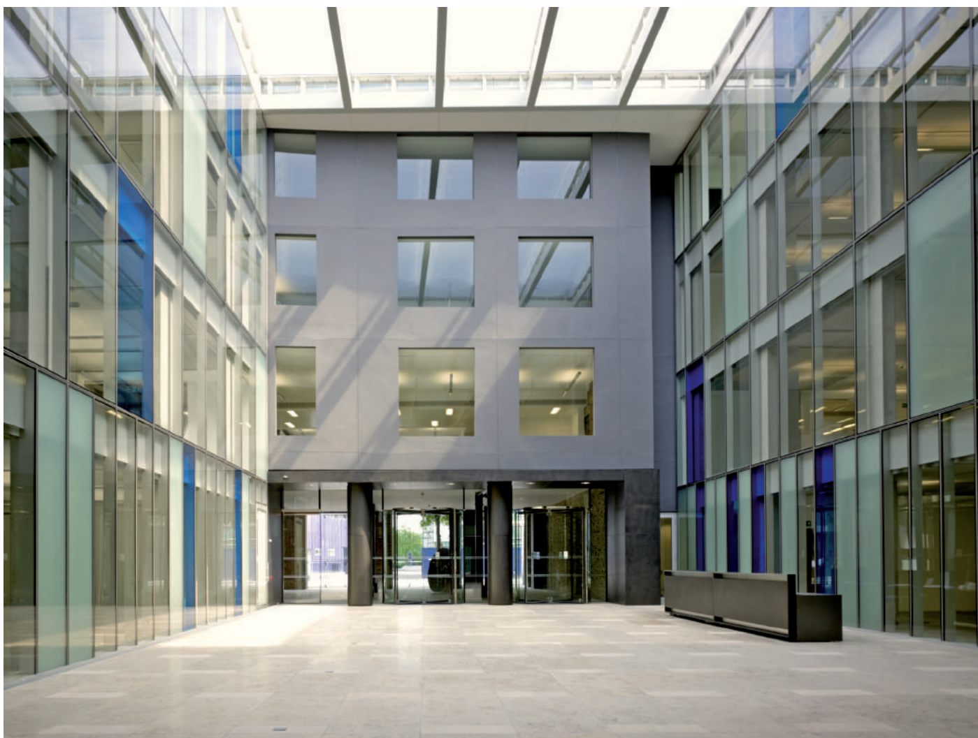
North wall of atrium
