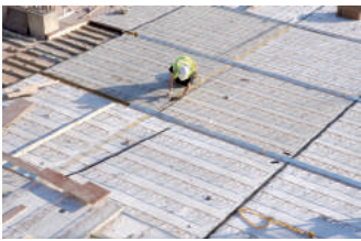
Precast biscuits being set out for pouring of slab
