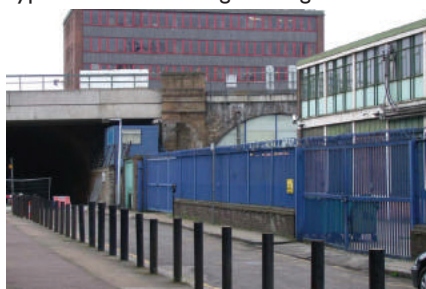
Barnham Street looking south
