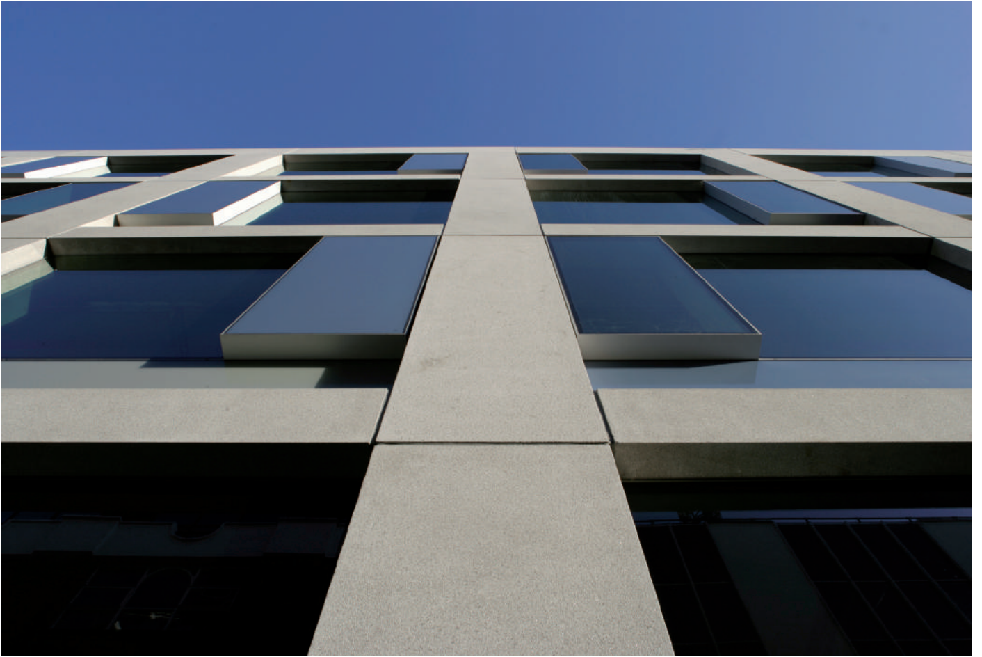
Site progress new build typical façade
