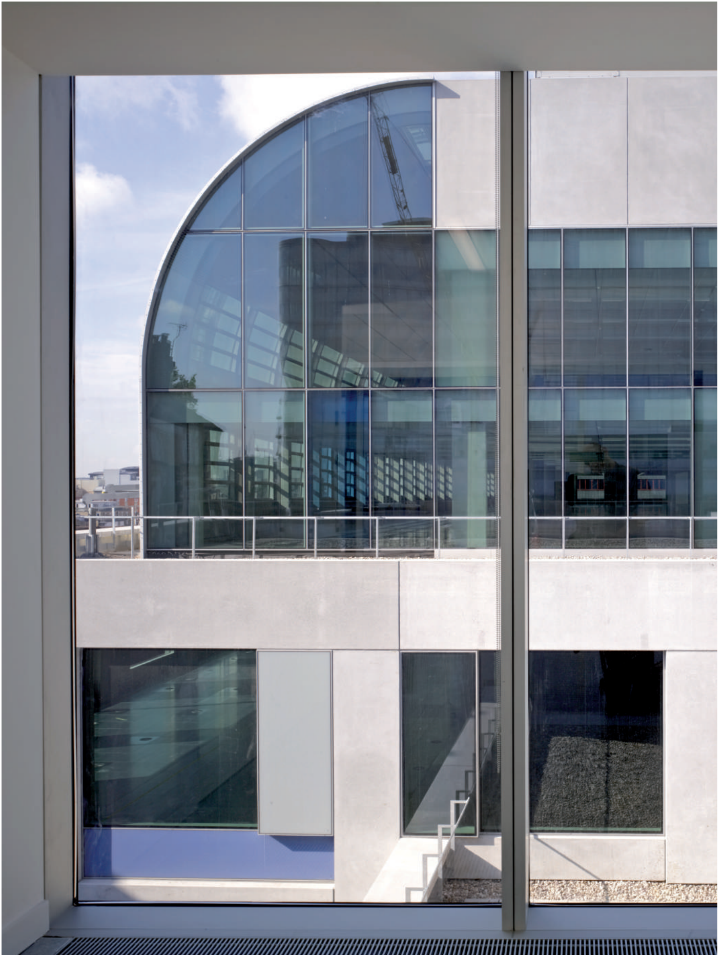
New build from Victorian building roof extension
