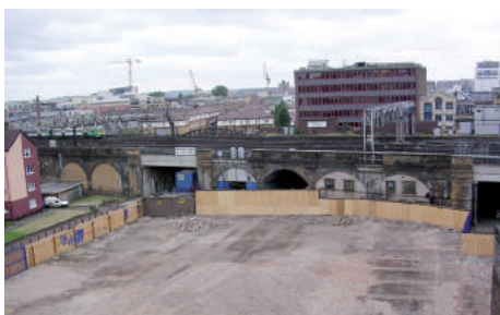
Cleared site looking south
