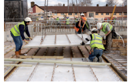
Crane lowering precast biscuit
