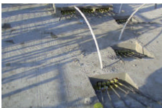
Post tensioning of slab
