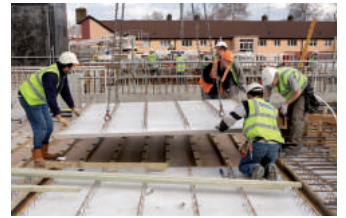
Crane lowering precast biscuit
