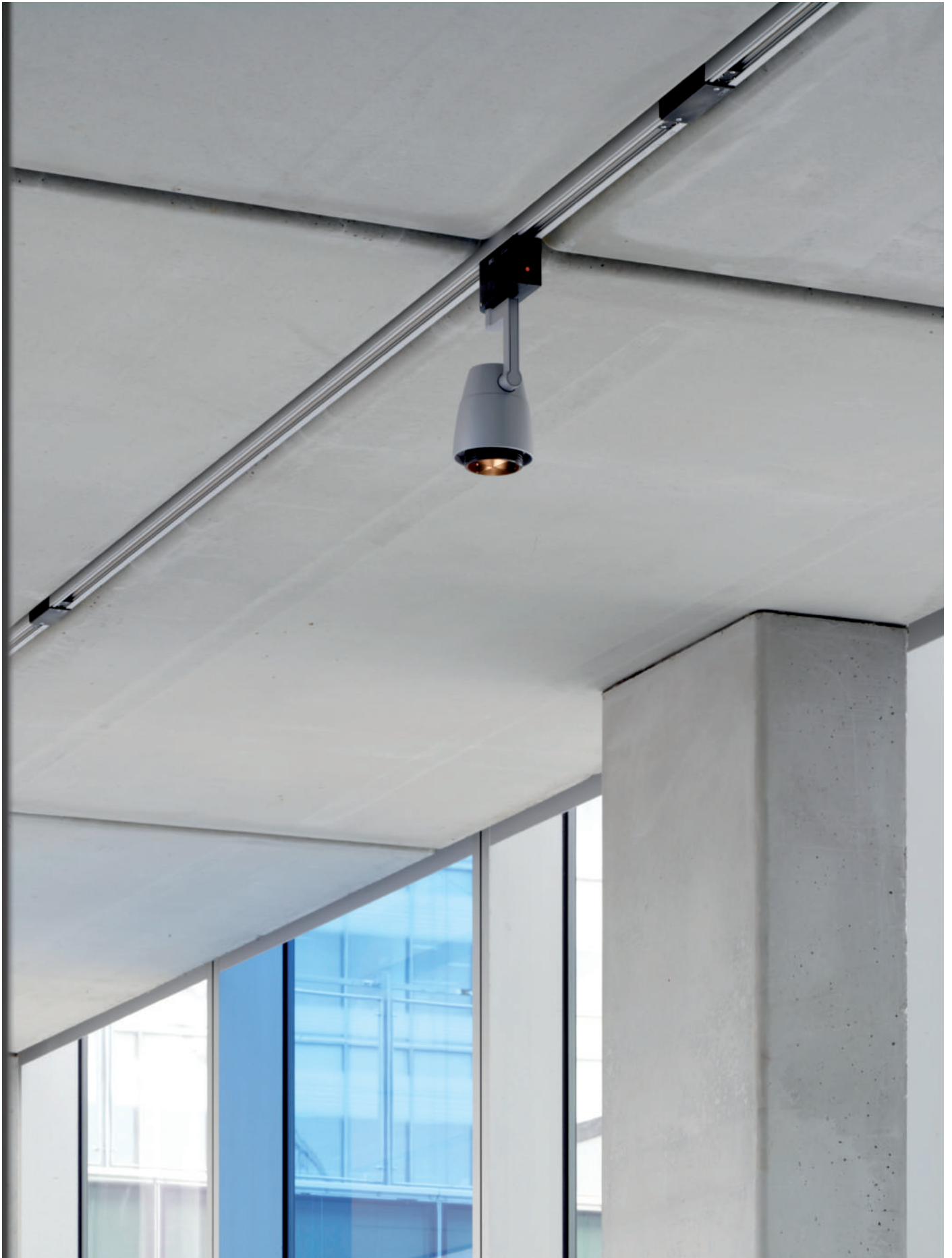
Pre-cast concrete soffit with atrium cladding behind
