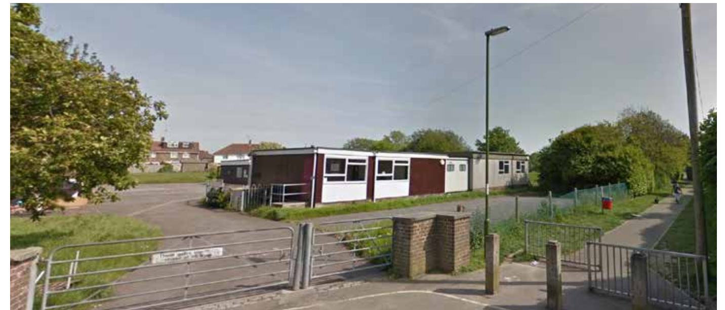
View of existing single storey education buildings 2014
