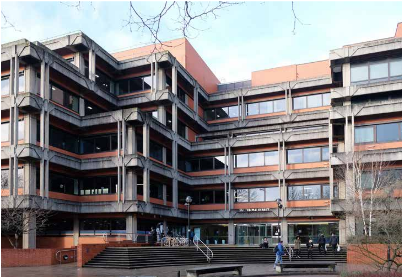
100 Temple Street main entrance
