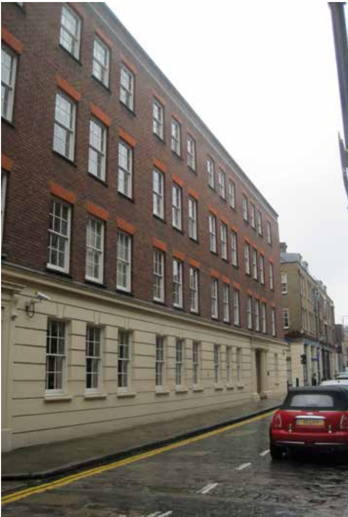
Existing view of Loom Court
