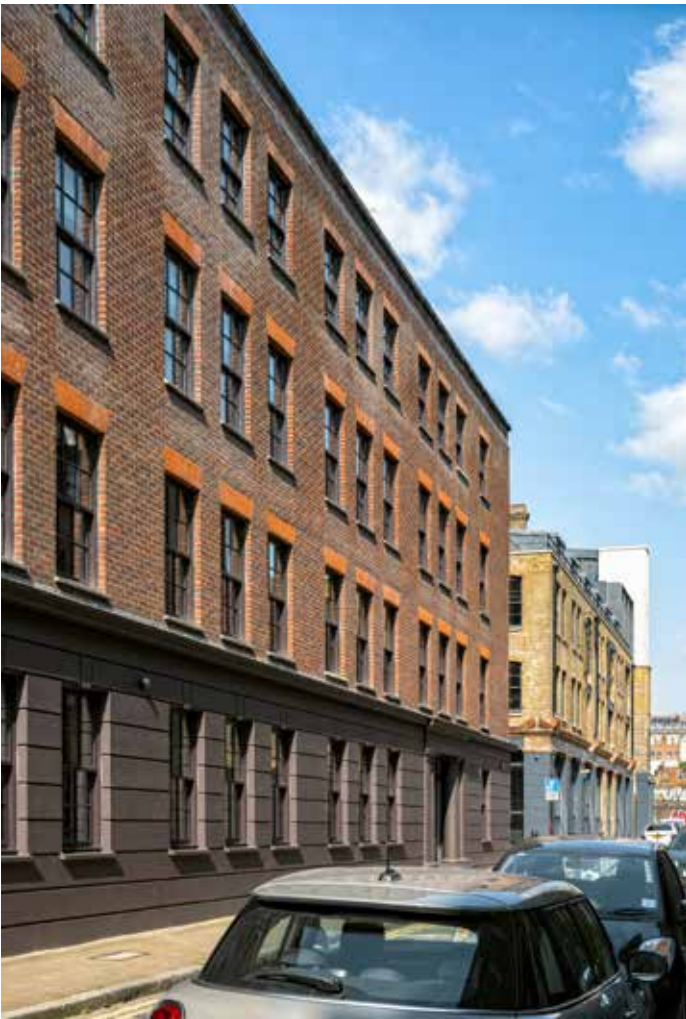
Refurbished elevations to Loom Court
