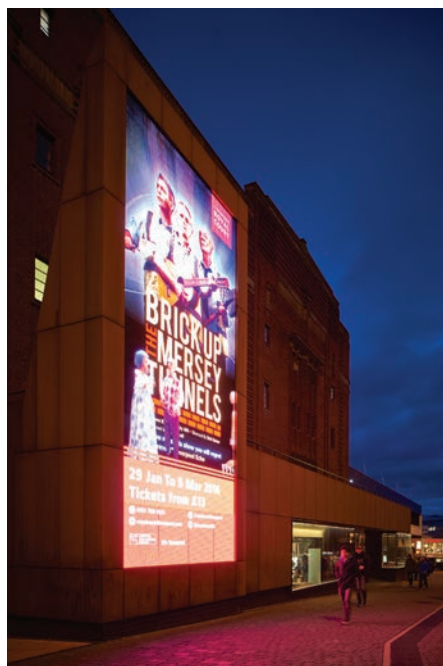
LED theatre signage incorporated into the new entrance extension (2)
