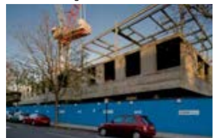
The structural frame nears completion
