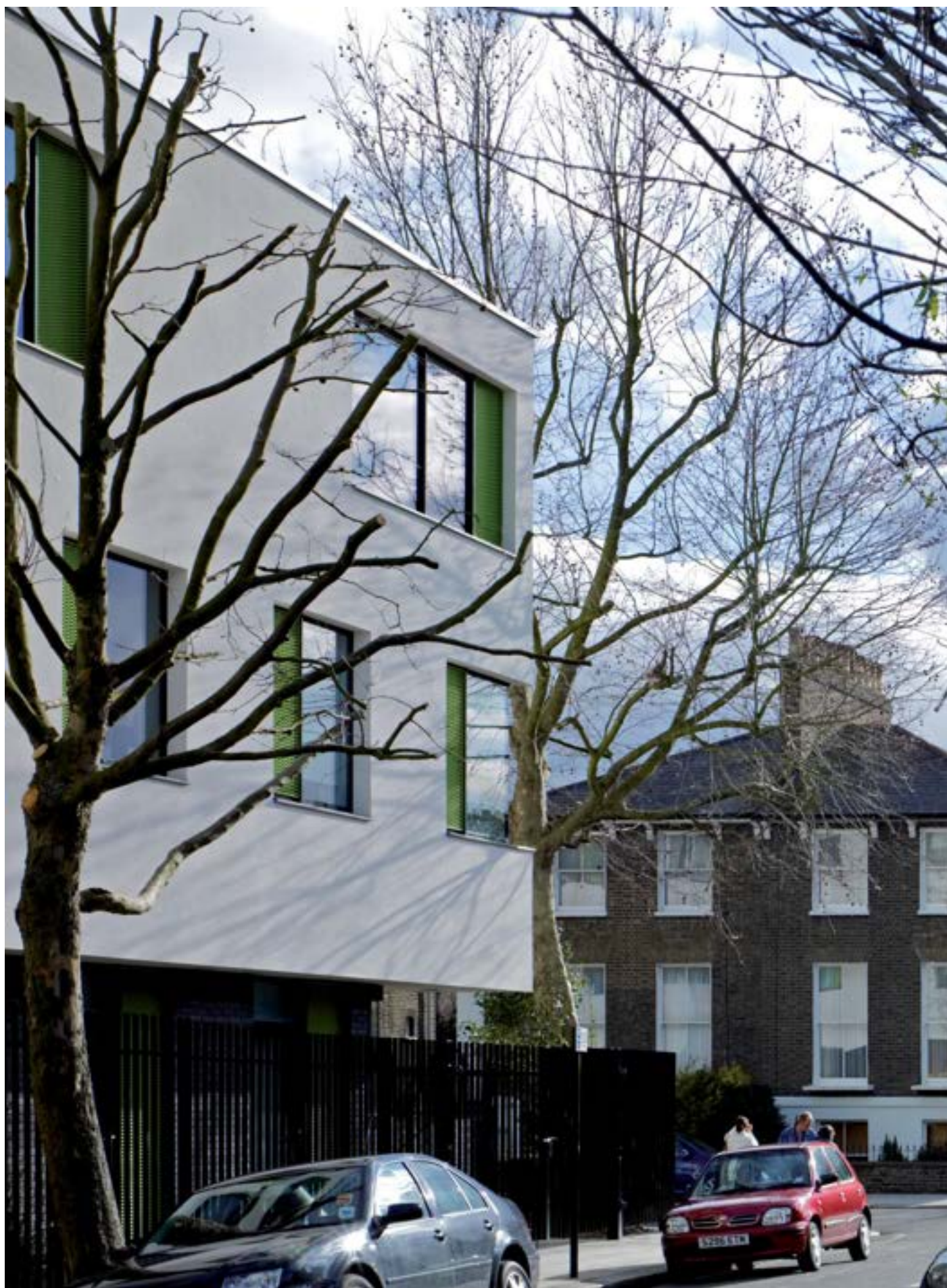
West Elevation at junction of Bartholomew Road and Bartholomew Villas
