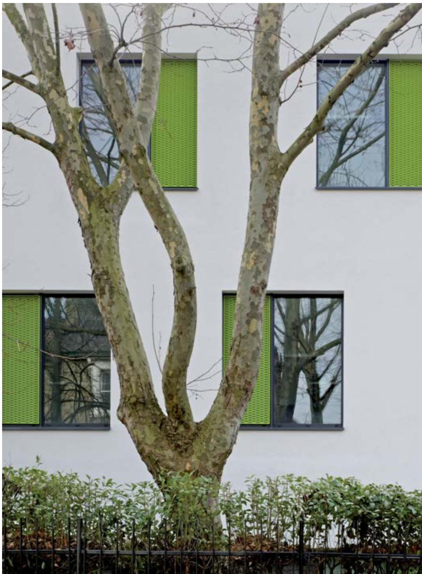
West Elevation fragment: Perforated grills to opening casement windows
