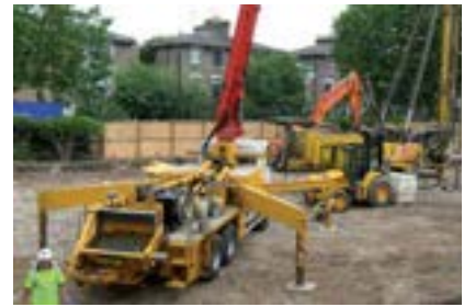
Piling is started on site
