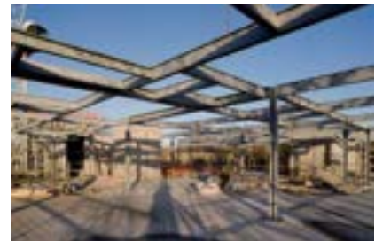
The roof is constructed in steel to reduce the loads on the large cantilevers
