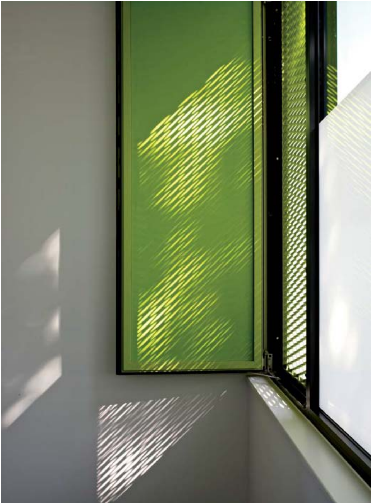
Typical East facing casement window that enables night time cool-
