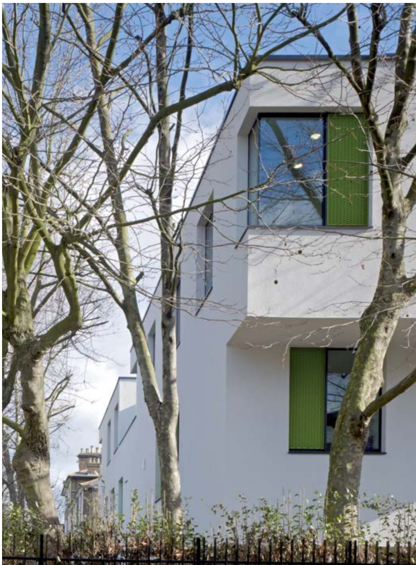
North West Corner
