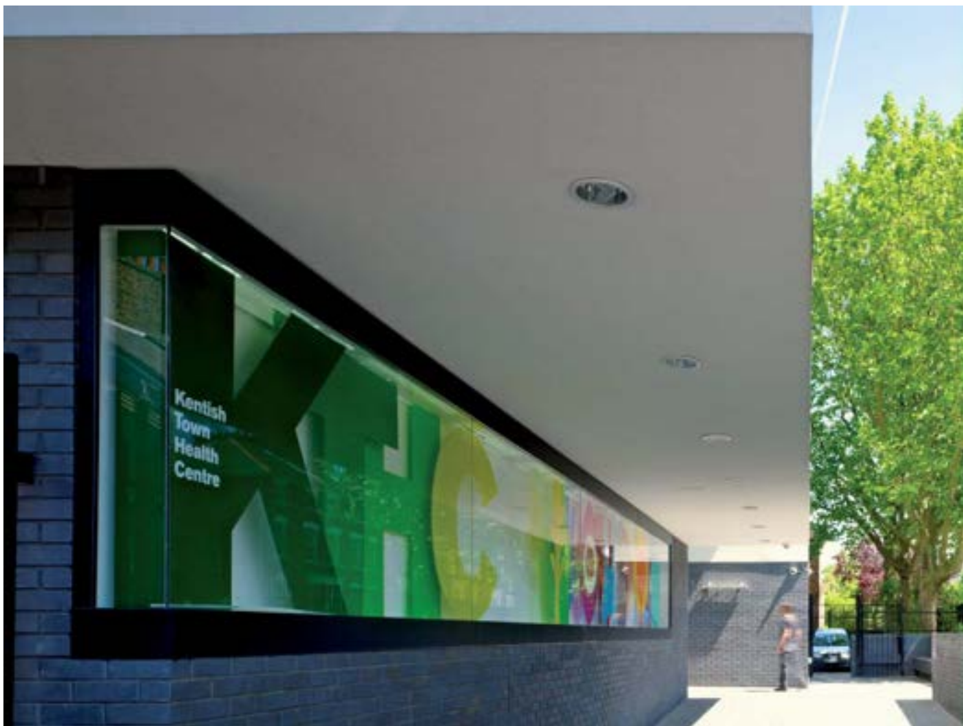
Light box under canopy leading to main entrance
