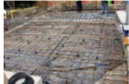
Ground floor slab is cast with heave protection below
