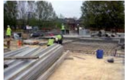
The second floor slab is cast. The floor plates act to tie the cantilever walls back to the stability cores
