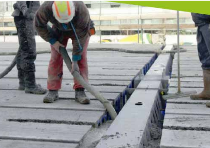
3 Pouring of concrete to set beam system
