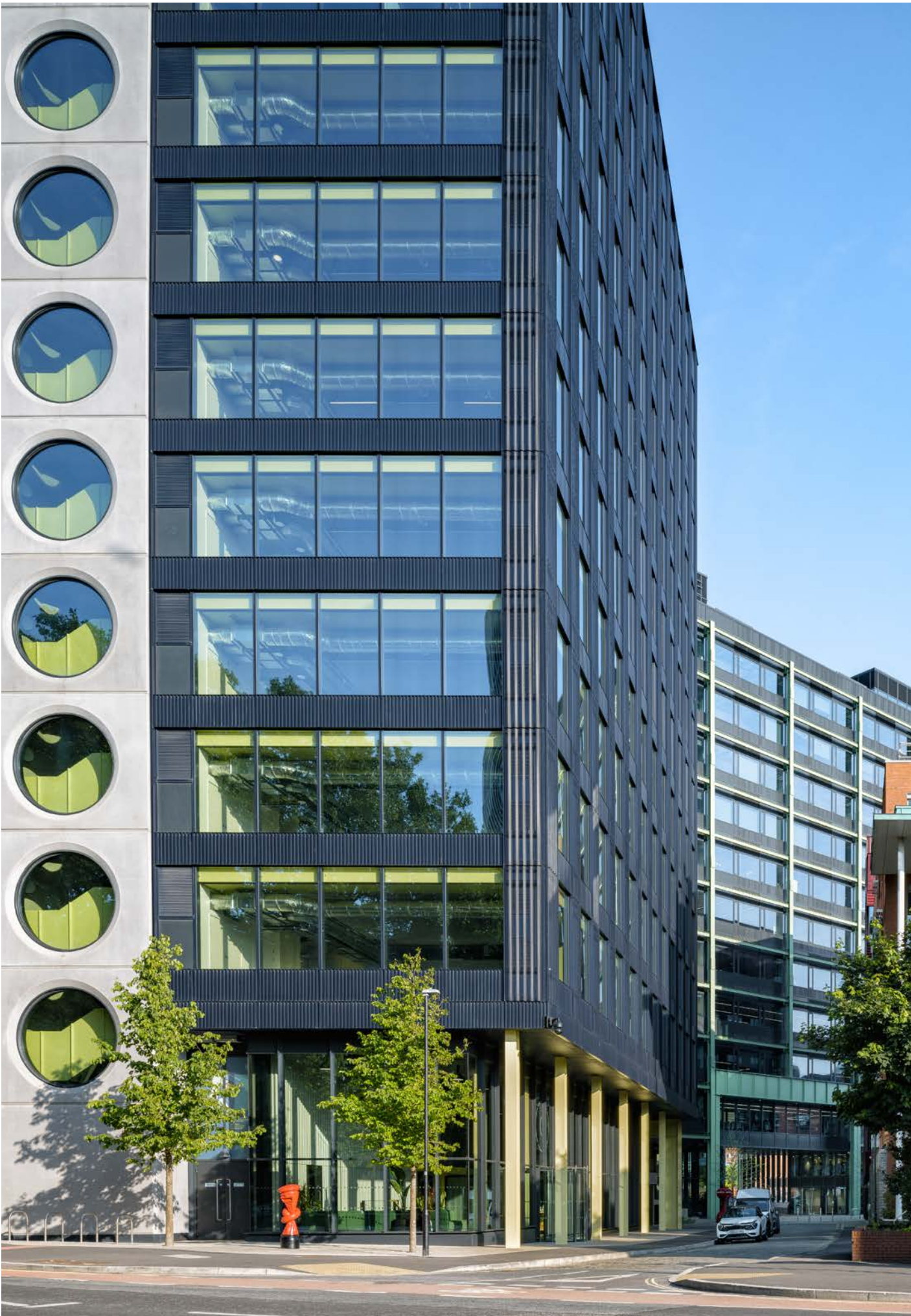
Reinstated entrance to campus along Cheese Lane - Tim Soar Photography
