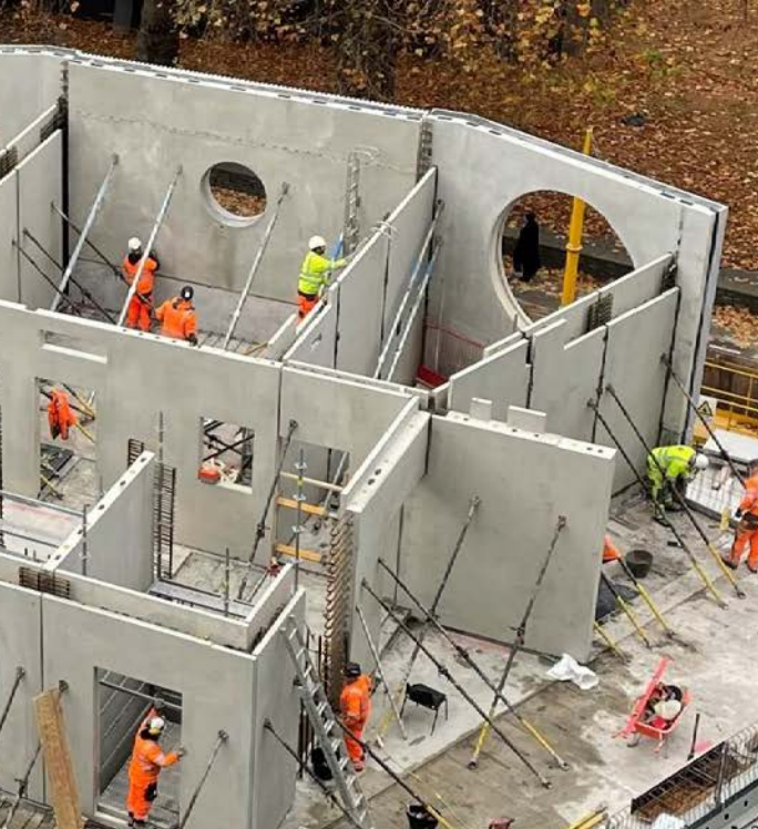
Precast Concrete Walls
