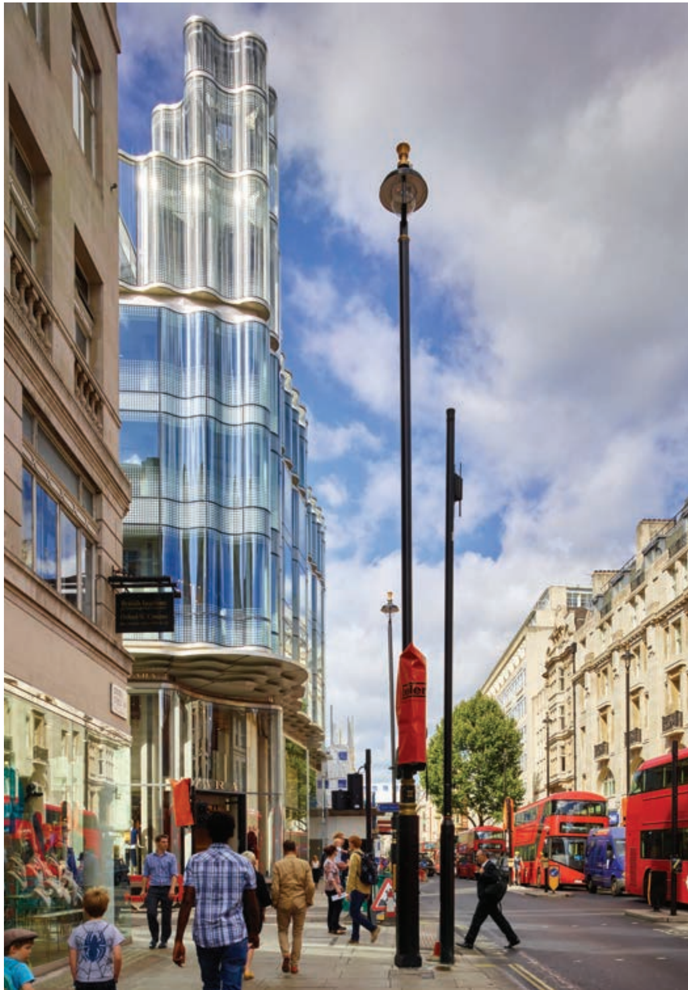
View looking west along Oxford Street
