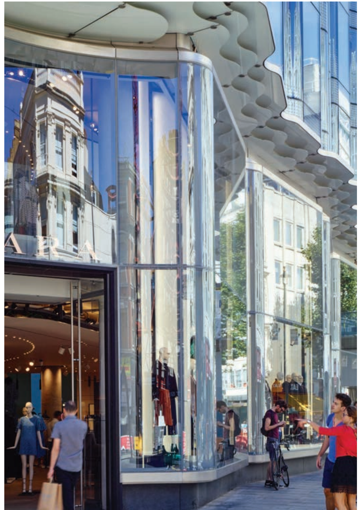
Detail of canopy and retail entrance
