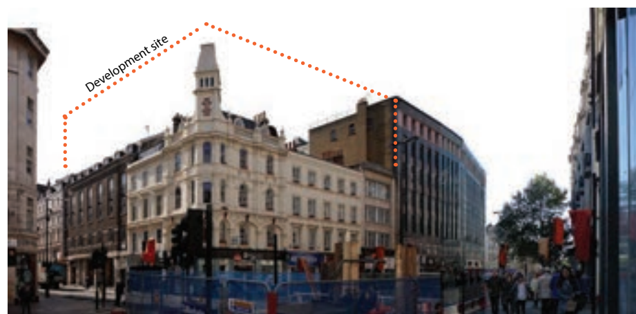
Development site showing disparate architectural styles, building heights and materials
